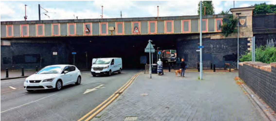
▲ ENHANCED ROUTE ALONG WEDNESFIELD ROAD
